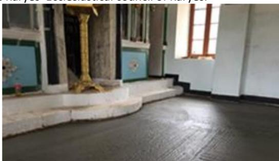
As you can see from the photos, after the serious problem in the foundations was repaired, the reconstruction of the floor was completed.
